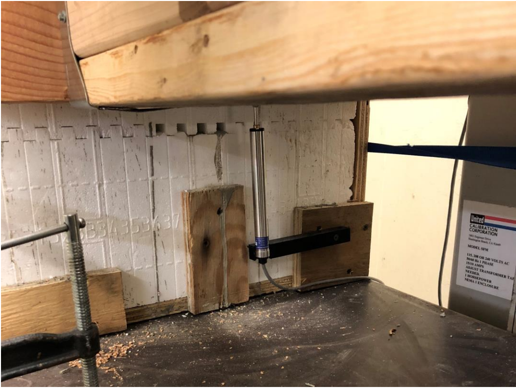
Figure 4. Test Setup- Left Joist Hanger
